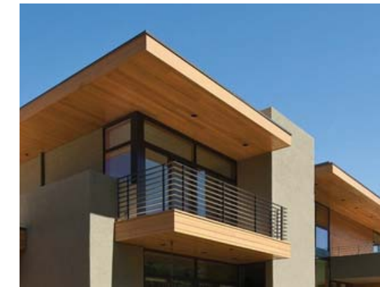
Ⓐ CEILING SOFFIT CONDITION
